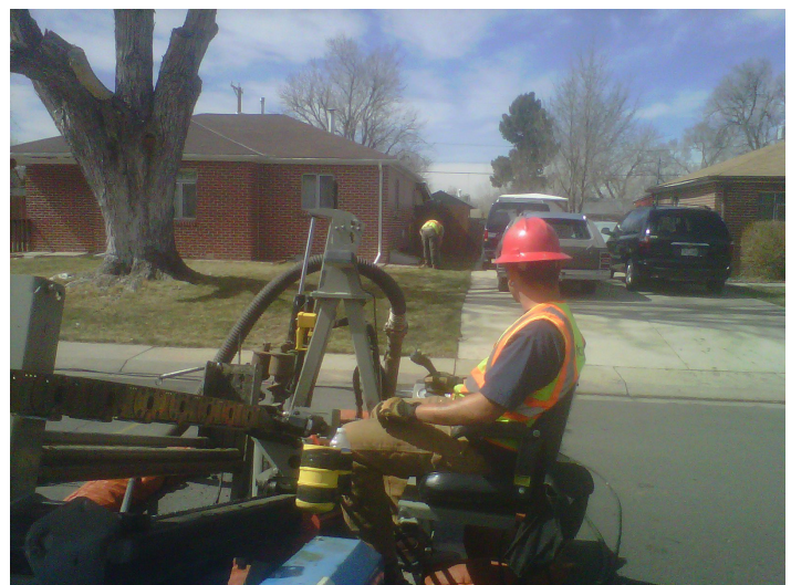
The Grundodrill 4X offers 9,800 lbs. of pullback and thrust.
