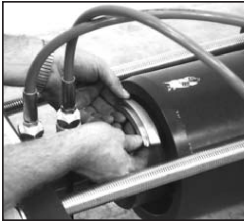
FIG. 58: INSTALL SEGMENT RING
