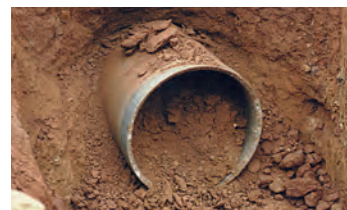
Casings are installed without surface slump.
